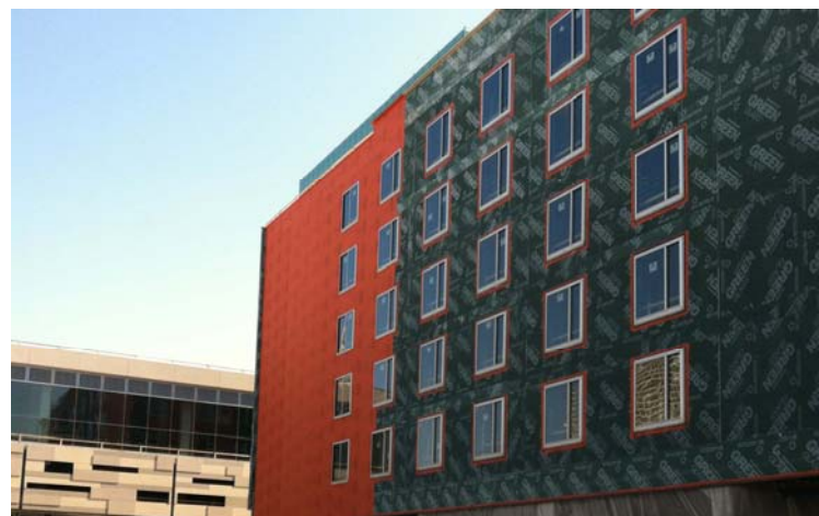
WrapShield SA Self-Adhered is tear, rip and puncture resistant during and after construction, thereby reducing repairs and labor costs.
