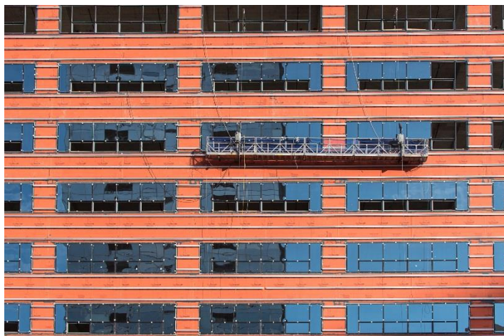
Modular panels used WrapShield SA SelfAdhered as part of their factory fabrication. The membrane was factory installed and the panels were transported to the site for installation.
