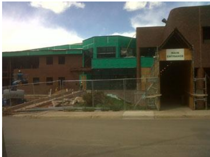
Over 7,000 sq.ft. of WallShield was installed at GC Energy.
