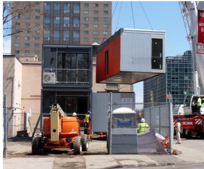
WrapShield SA Self-Adhered Water Resistive Vapor Permeable Air Barrier Sheet (orange) provides superior protection on NYC’s Post-Disaster Housing Prototype. Photo courtesy of Mary Frost.
