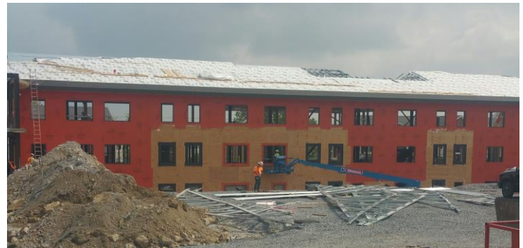
WrapShield SA Self-Adhered (orange) was chosen for its exceptional drying capacity and ability to be applied in low temperatures.
