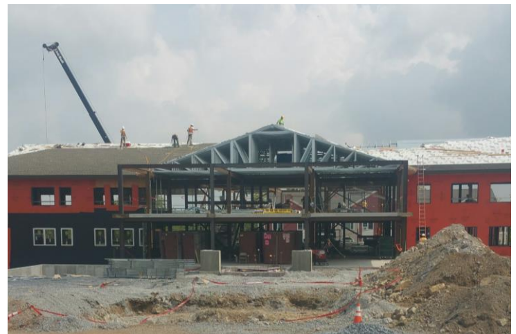
WrapShield SA Self-Adhered (orange) was chosen for its exceptional drying capacity and ability to be applied in low temperatures.
