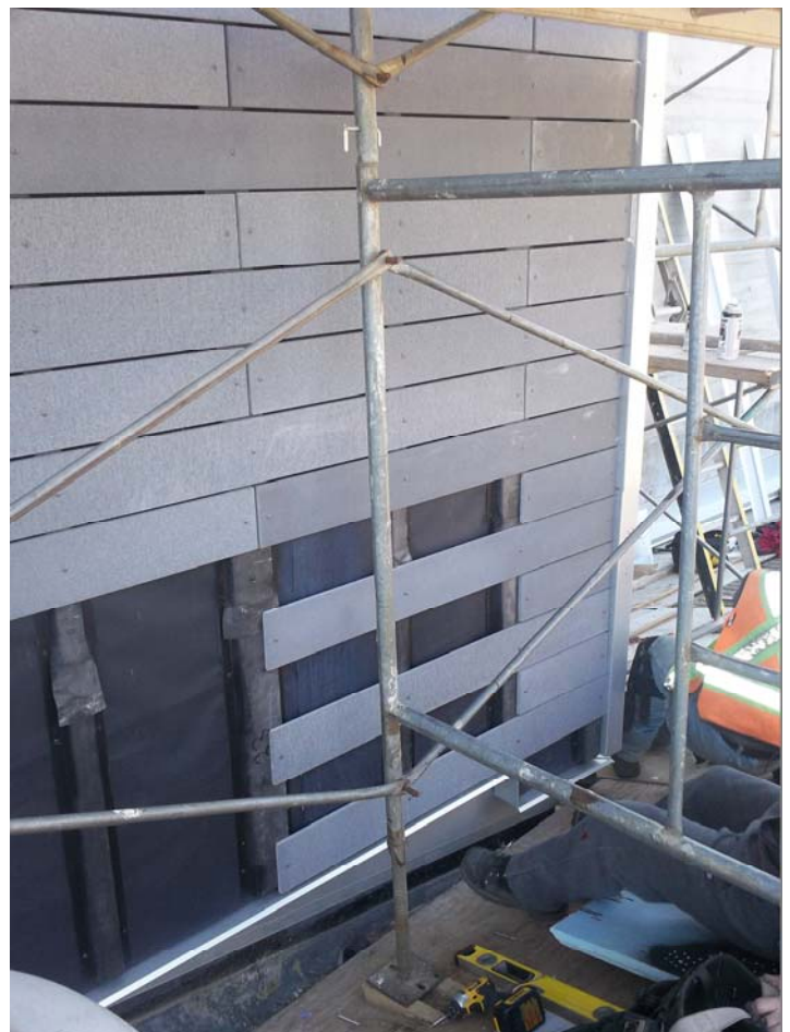
RevealShield combines the best properties of a water resistive highly vapor permeable air barrier and black UV resistant sheet membrane into one product for open joint cladding systems.
