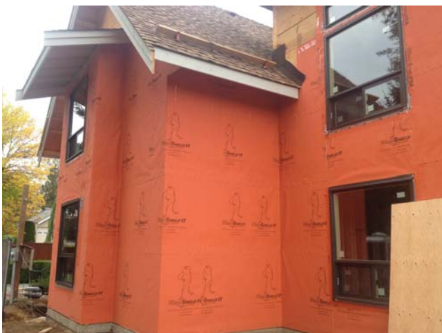
(below) WrapShield Water Resistive Vapor Permeable Air Barrier membrane construction.
