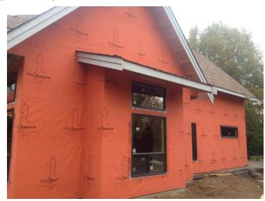
Over 4,000 sq. ft. (1,219 M²) of WrapShield and WrapShield SA Self-Adhered Air Barrier is installed on a private residence in Langely, British Columbia.
