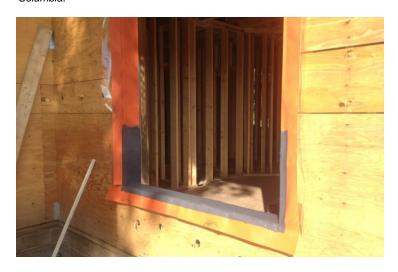
(above) VaproLiqui-Flash (gray) liquid applied waterproof flashing material is applied around the rough opening of a window.
