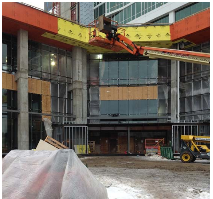
Approximately 21,378 sq. ft. of WrapShield SA Self-Adhered Air Barrier (orange) installed on Potawatomi Bingo Casino.
