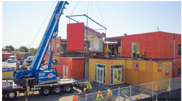
The modules were brought in by crane to their final positions at Educare of Los Angeles at Long Beach .
