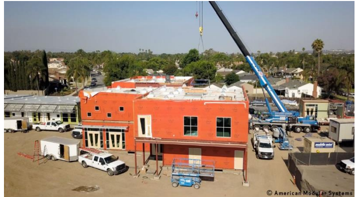
WrapShield SA Self-Adhered WRB/Air Barrier (orange) was installed on 9 modules at the American Modular Systems factory in Manteca, CA before being delivered to their final location in Long Beach, CA.
