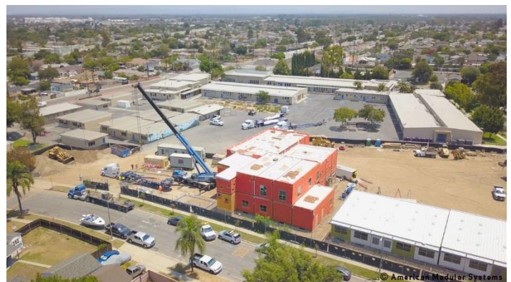
WrapShield SA Self-Adhered's ability to be exposed for up to six months was instrumental in accommodating the characteristic shipping process of modular construction.
