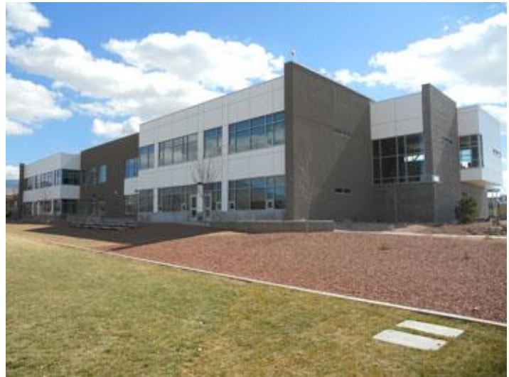
Over 10,000 sq.ft of VaproShield Wrapshield was used on the high school.
