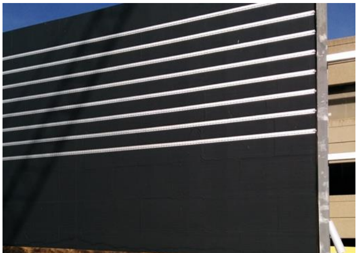
This highly vapor permeable, UV stable, open joint rainscreen cladding system created a durable, sustainable building that provides a healthy indoor environment
