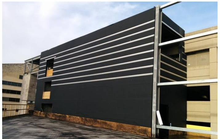
RevealShield contains zero VOC's, provides exceptional UV stability for open joint cladding, and requires no special installation equipment.
