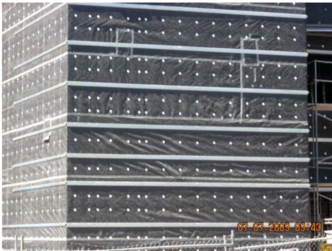
90,000 ft2 of Wrapshield Black was used on the expansion of the Crocker Art Museum.
