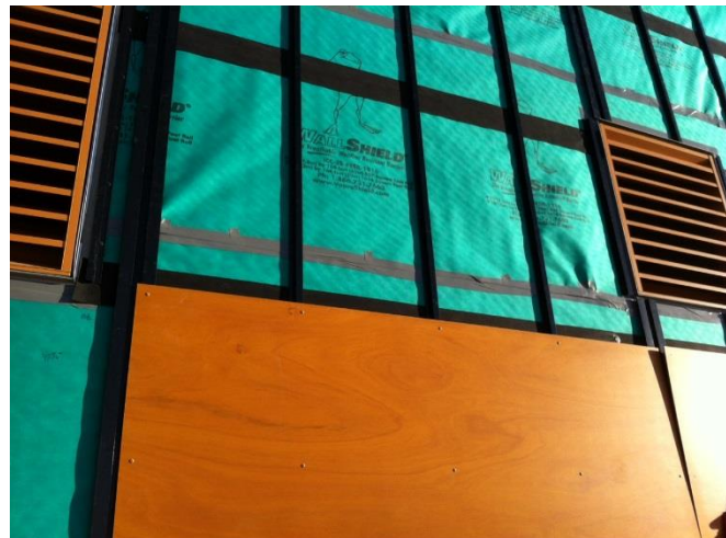
WallShield and WrapShield Black offer UV protection and temperature resistance during installation.
