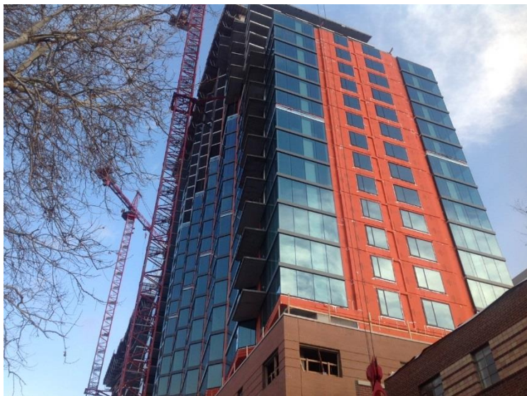
WrapShield SA Self-Adhered WRB/Air Barrier (orange) is being installed on The Country Club Towers in Denver, Colorado.
