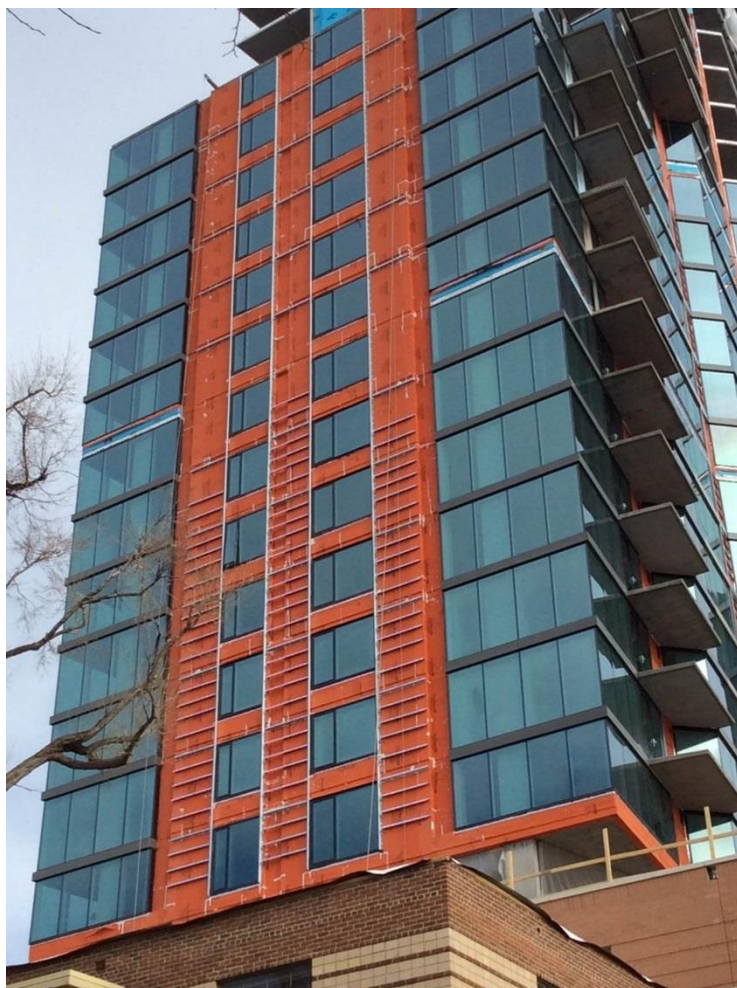
WrapShield SA Self-Adhered does not require any primer, and crews are always safe around the product as it emits zero VOC's and contains no red list chemicals.
