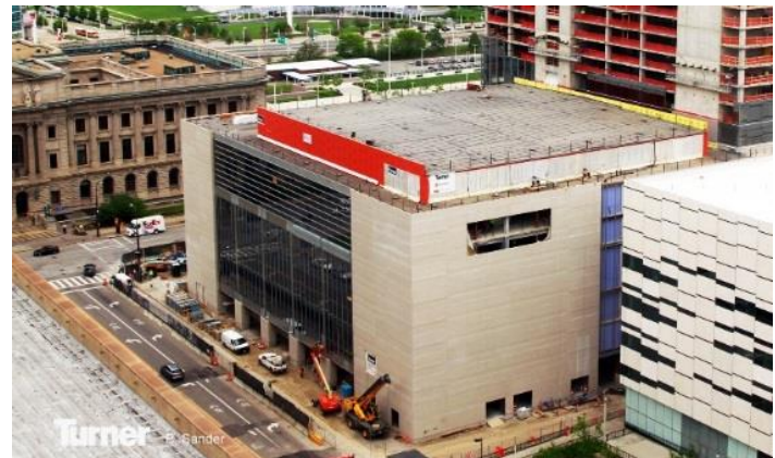
WrapShield SA can withstand up to 6 months of direct exposure to elements such as wind, rain and snow.
