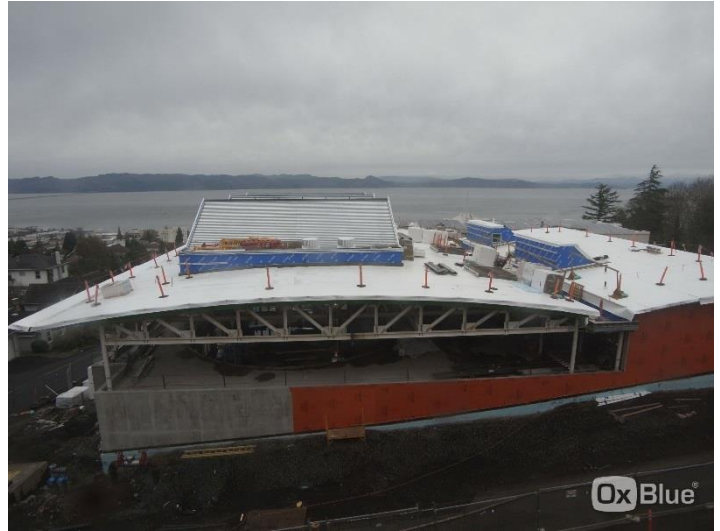
WrapShield SA Self-Adhered (orange) WRB/Air Barrier easily adhered to multiple substrates- including CIP concrete and gypsum sheathing—despite the damp climate and challenging schedule.
