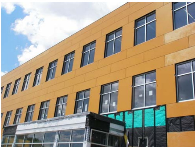
WallShield was installed behind 44,000 ft2 of Trespa.
