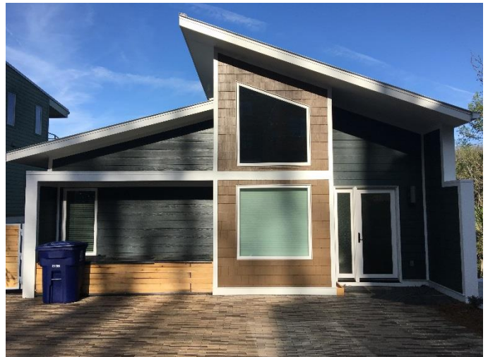
WrapShield IT Integrated Tape was installed behind an open joint mixed façade of fiber cement rain screen cladding and wood.
