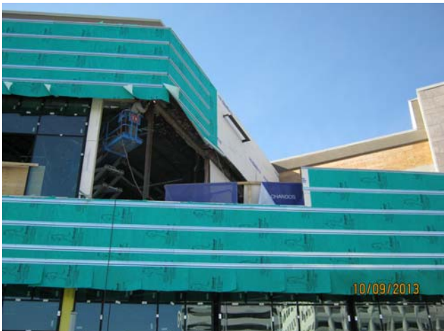
WallShield installs easily and can span framing members without solid substrate providing moisture protection and facilitating completion of the "dry-in" phase.
