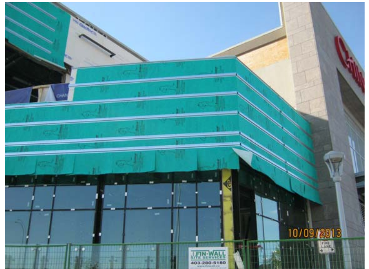
WallShield installs easily and can span framing members without solid substrate providing moisture protection and facilitating completion of the "dry-in" phase.
