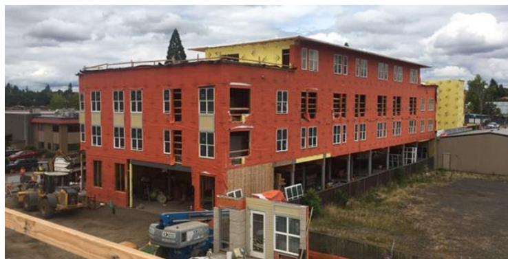
*Rough openings on the Burnham & Ash Apartments were flashed using pre-cut field membranes; VaproFlashing.*
