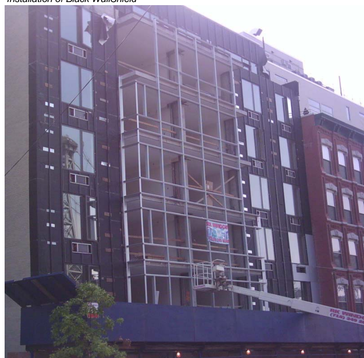
View of Black WallShield installation from across the street
