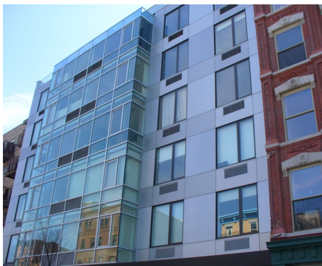
Completed in 2007 the Bridgeview Towers in Brooklyn, NY Trespa panels over Black WallShield
