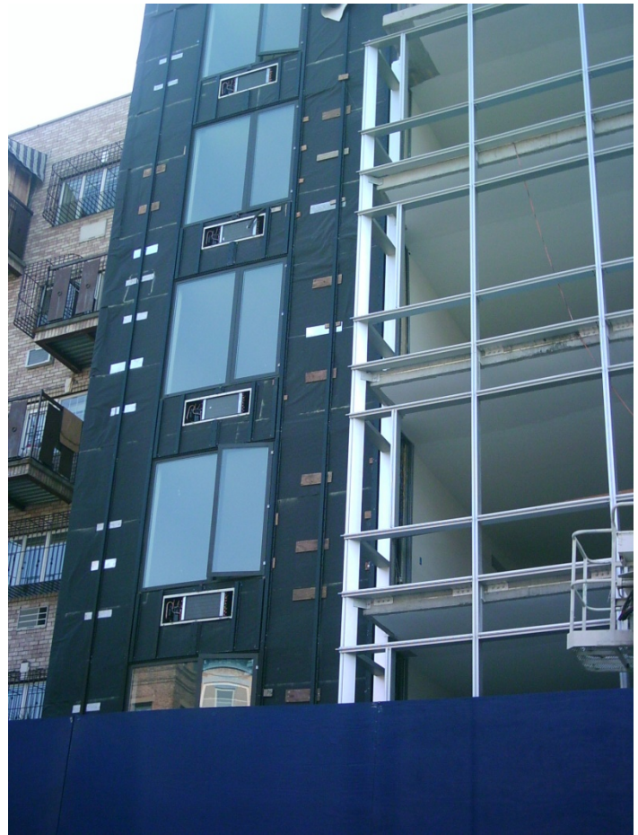
Installation of Black WallShield
