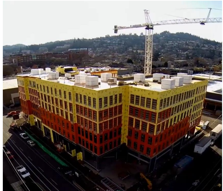
Slabtown Market switched to WrapShield IT Integrated Tape WRB/AB, citing the product's durability and ability to be installed in wet weather compared to the originally specified liquid-applied barrier.
