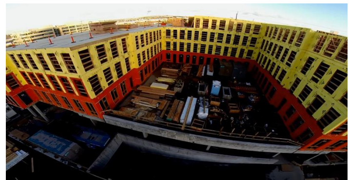
VaproShield WRB/AB membranes easily accommodated the multiple types of exterior veneers used in this complex renovation.
