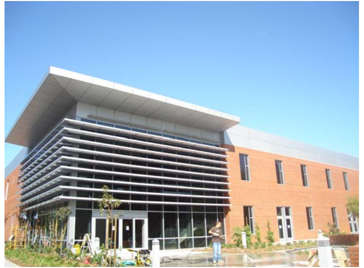
The main entrance of Biola University Crowell School of Business. Trespa panels created exposed areas of the building envelope therefore WallShield was used to protect exposed areas from UV, mold and mildew.
