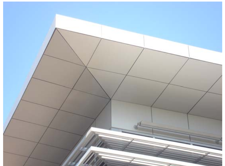
Up close view of the Trespa panels.
