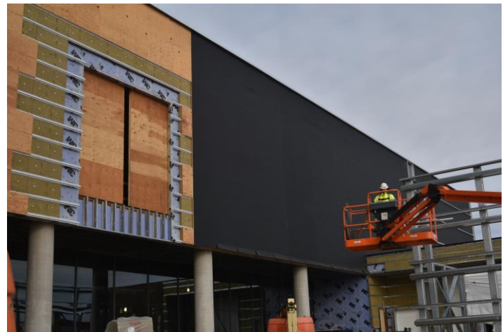
RevealShield SA Self-Adhered eliminates the need for time intensive substrate and rough opening preparation—saving labor costs and time.
