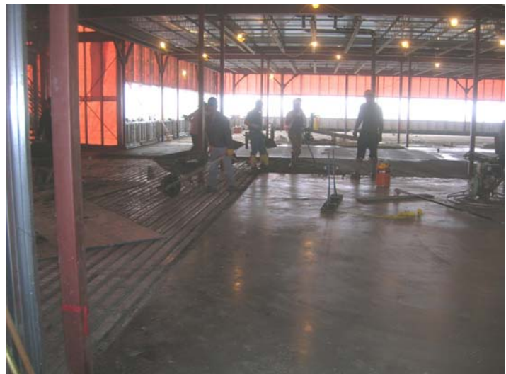
Structure enclosed with WrapShield (orange) allowing interior construction to continue. 6/25/06
