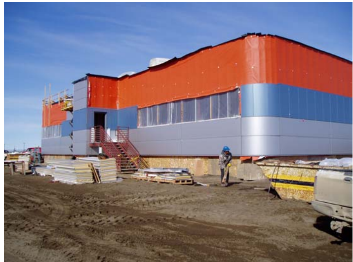
Structure enclosed with WrapShield (orange) allowing interior construction to continue. 6/25/06
