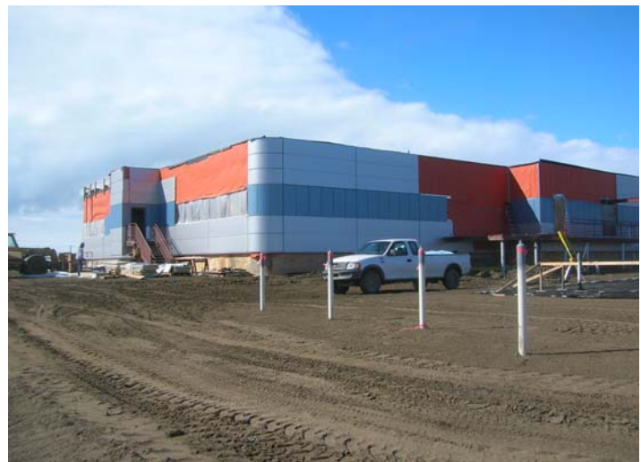
Phase I nearly enclosed, showing VaproShield's WrapShield (orange) 7/16/2006
