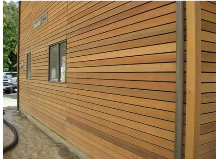
Detail of open joint rain screen design Prodemia cladding with VaproFlashing Black
