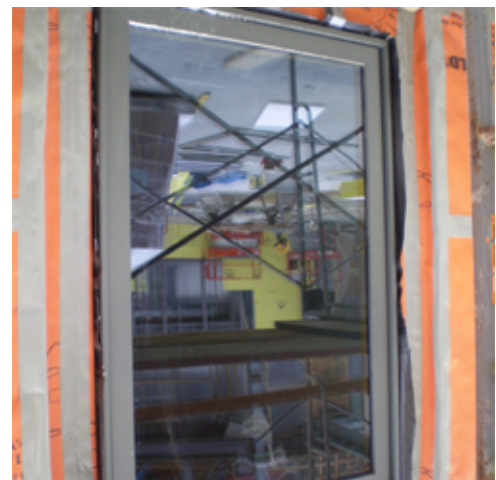
Window after installation.
