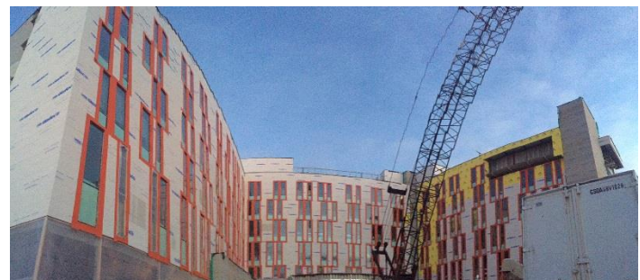
VaproFlashing (orange), which quickly dried in the building, was used around the window rough openings, allowing glazing to be installed before the siding, keeping trades on schedule
