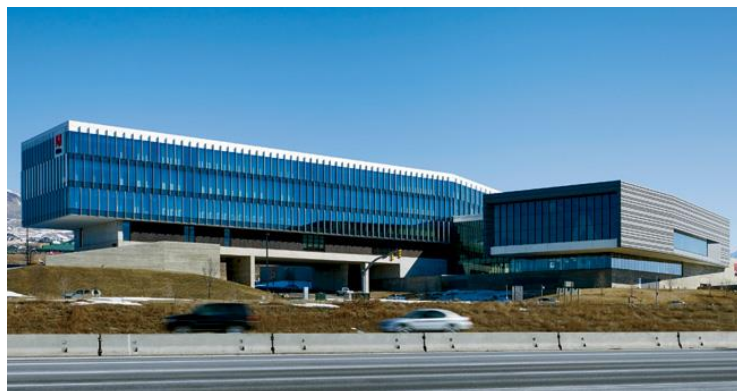
Image courtesy of © Tim Griffin Architectural Record Magazine, Sept. 2013 WrapShield SA Self-Adhered was installed behind steel-and-glass façade.
