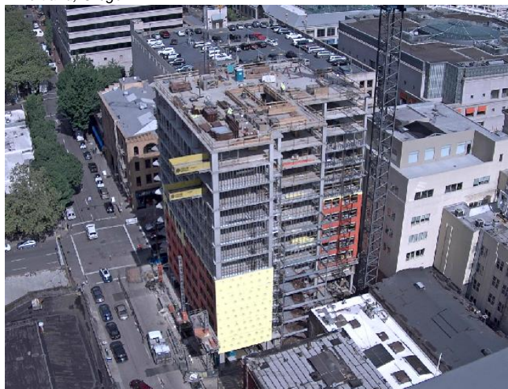
Approx. 40,000 sq.ft. of WrapShield SA Self-Adhered (orange) WRB/Air Barrier is being installed on the new AC Hotel by Marriott in Portland, Oregon.
