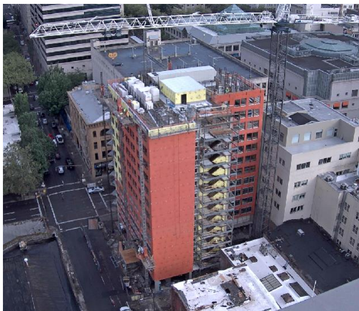
Approx. 40,000 sq.ft. of WrapShield SA Self-Adhered (orange) WRB/Air Barrier is being installed on the new AC Hotel by Marriott in Portland, Oregon.
