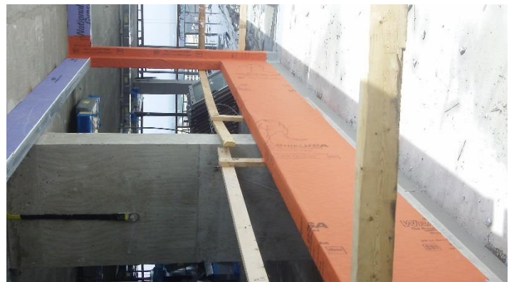
WrapShield SA Self-Adhered Water Resistive Vapor Permeable Air Barrier Sheet Membrane served as an in-process replacement on Eleven 55 Ripley after the original fluid-applied air barrier failed to withstand the cold Maryland weather.
