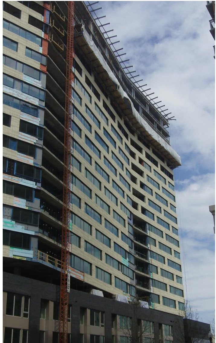
WrapShield SA Self-Adhered Water Resistive Vapor Permeable Air Barrier Sheet Membrane served as an in-process replacement on Eleven 55 Ripley after the original fluid-applied air barrier failed to withstand the cold Maryland weather.
