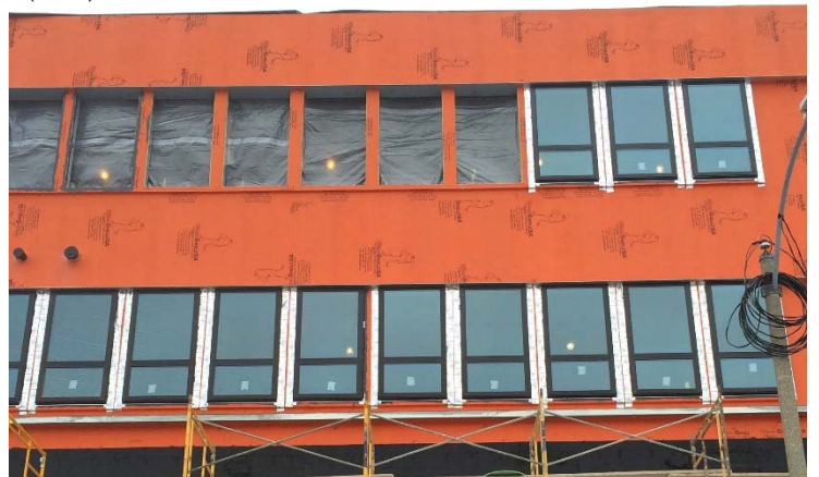
WRAPSHIELD SA ® SELF-ADHERED combines the best properties of a vapor permeable membrane and air barrier in one innovative, affordable self-adhering product.
