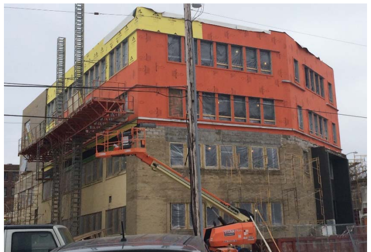
WRAPSHIELD SA ® SELF-ADHERED is applicable for all climates and weather conditions, and can be installed in temperatures as low as 20°F (-6° C)
