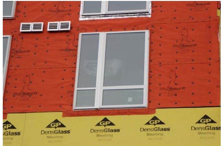
Rough openings were sealed using VaproFlashing and VaproLiqui-Flash.
