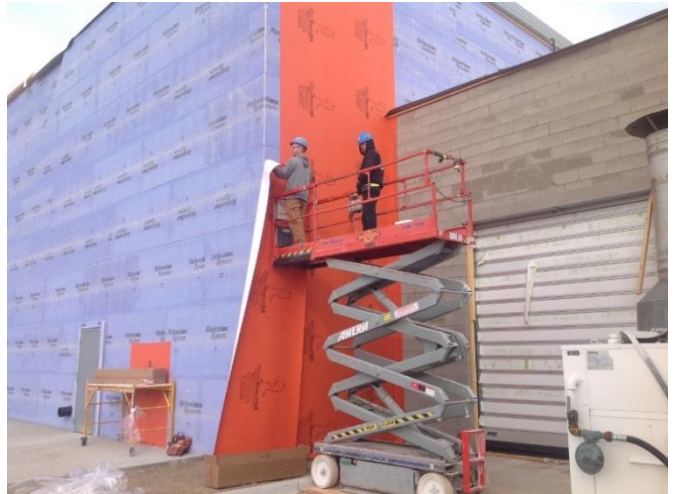
Installers use basic handtools to efficiently install WrapShield SA Self-Adhered (orange) over over cement block and gypsum sheathing. The packaging box serves as a dispenser.
