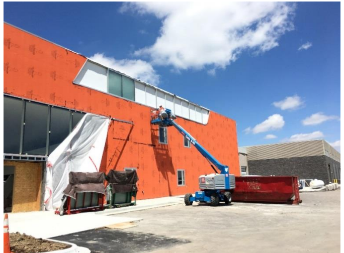
WrapShield SA Self-Adhered does not require any primer, and crews are always safe around the product as it emits zero VOC's and contains no red list chemicals.
