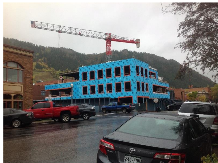
WrapShield SA Self-Adhered is phase construction friendly allowing installation for all climates and weather conditions.
