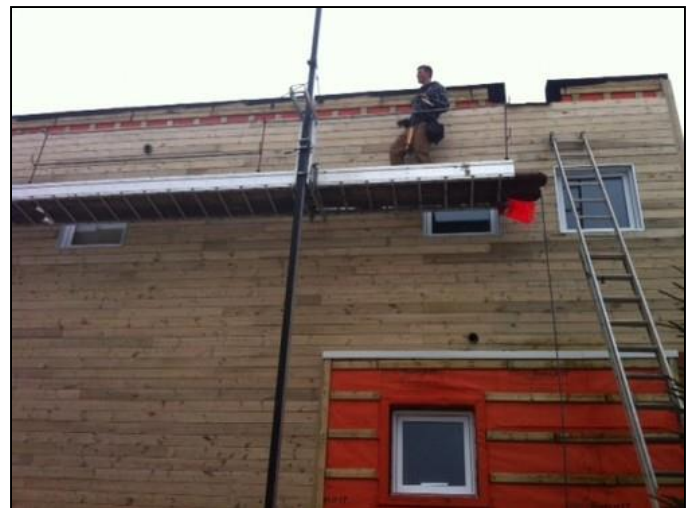
WrapShield Water Resistive Vapor Permeable Air Barrier Membrane was installed.
