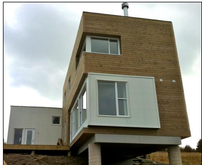
Home after completion.
