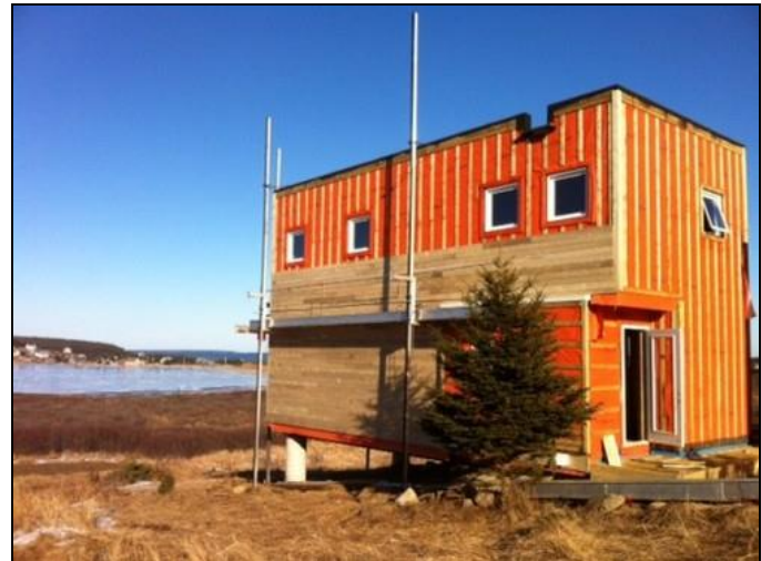
WrapShield Water Resistive Vapor Permeable Air Barrier Membrane was installed.
