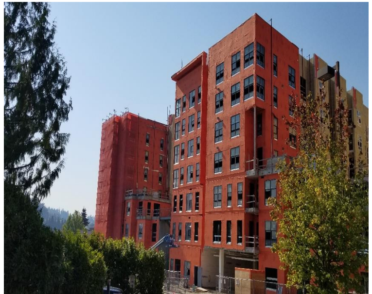
WrapShield SA helps protect the delicate building envelope by reducing moisture intrusion and preventing mold, mildew and rot in the moist cold climate of the Pacific Northwest.
