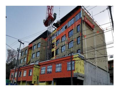
WrapShield helps reduce energy costs, reduces noise, and protects the delicate building envelope from moisture intrusion and mold, mildew and rot in the moist cold climate of the Pacific Northwest.
