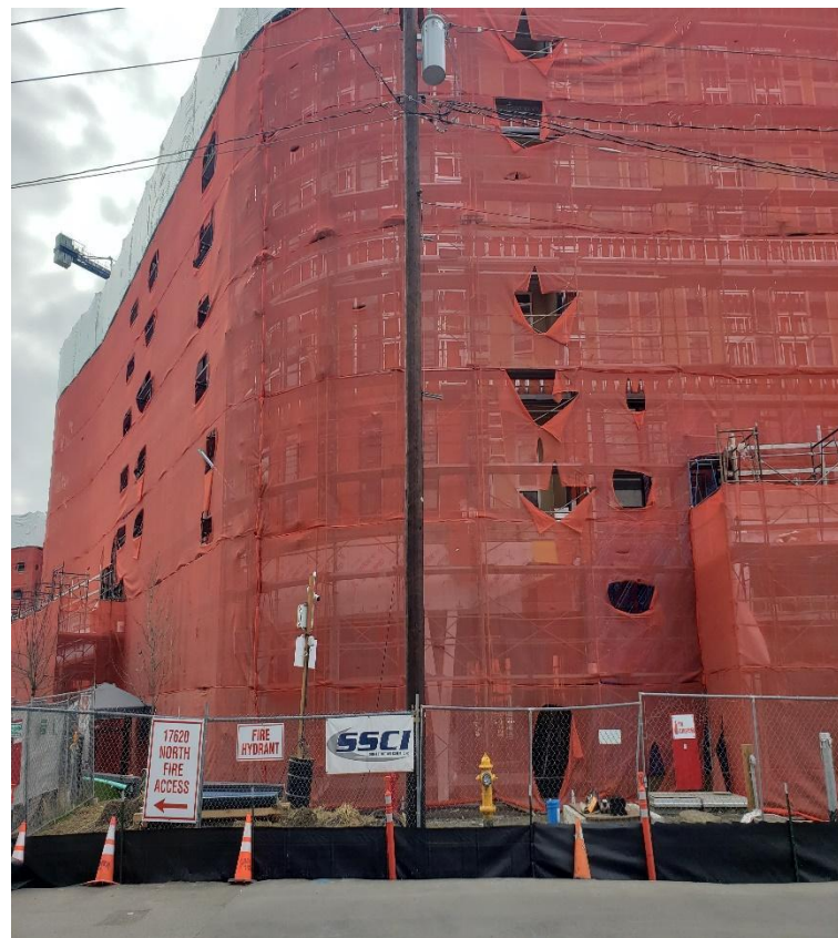
WrapShield helps protect the delicate building envelope by reducing moisture intrusion and preventing mold, mildew, and rot in the moist cold climate of the Pacific Northwest.
