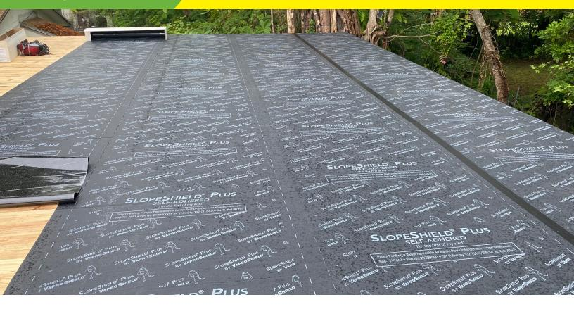
Over 3,500 sq.ft. of SlopeShield Plus Self-Adhered (SA) vapor permeable roofing underlayment was used in the first cross-laminated timber (CLT) project, Grovehaus, in Miami, Florida. In addition, 3,300 sq.ft. of PanelShield SA, a permeable polyester air barrier WRB membrane, was used on the exterior walls in this mass timber build.
