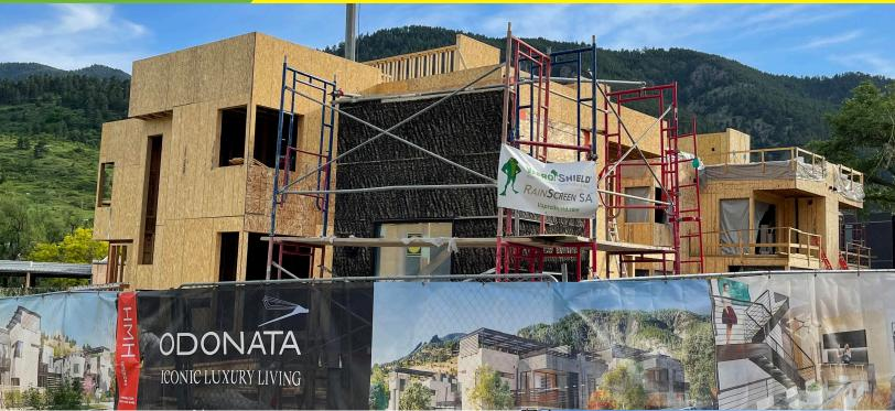
Over 60,000 sq. ft. of RainScreen SA was installed on the Odonata luxury condominiums located in Boulder, CO. RainScreen SA, self-adhered air and water resistive barrier with factory installed drainage matrix will reduce the incidence of moisture related damage behind the cladding system by creating an essential drainage plane allowing moisture to move away from the structure.
