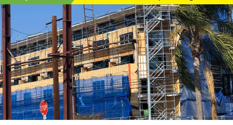
Over 5,800 sq. ft. of VaproShield products, including RainScreen SA self-adhered Air Barrier (AB) Water Resistive Barrier (WRB) with built-in rainscreen drainage matrix were installed on a West Los Angles, California multi-family housing build. RainScreen SA's new aggressive adhesive bonded without primer to the OSB substrate used in this project.
