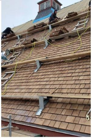
SlopeShield Plus roofing underlayment installed under cedar shakes.
