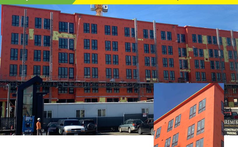
WrapShield SA Self-Adhered was installed on Saltwood North and South, a 354-unit, mixed-use development stretching across a block of Portland's vibrant Slabtown neighborhood.
