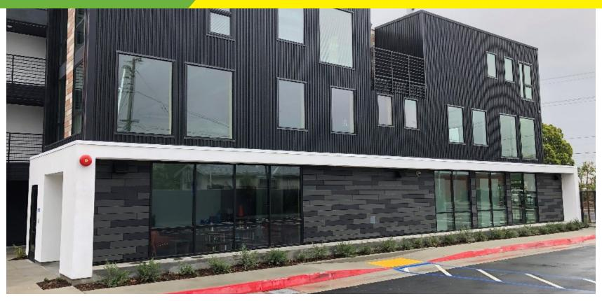
13,000 sq. ft. of RevealShield SA Self-Adhered was installed on the brand-new Carson Arts Colony under modern and colorful open-joint fiber cement panels, with VaproLiquiFlash installed at the building's penetrations. As the design incorporated perforated metal panels, the architect needed an air & water-barrier that was UV-stable and would not deteriorate in sunlight like so many water-barriers do.
