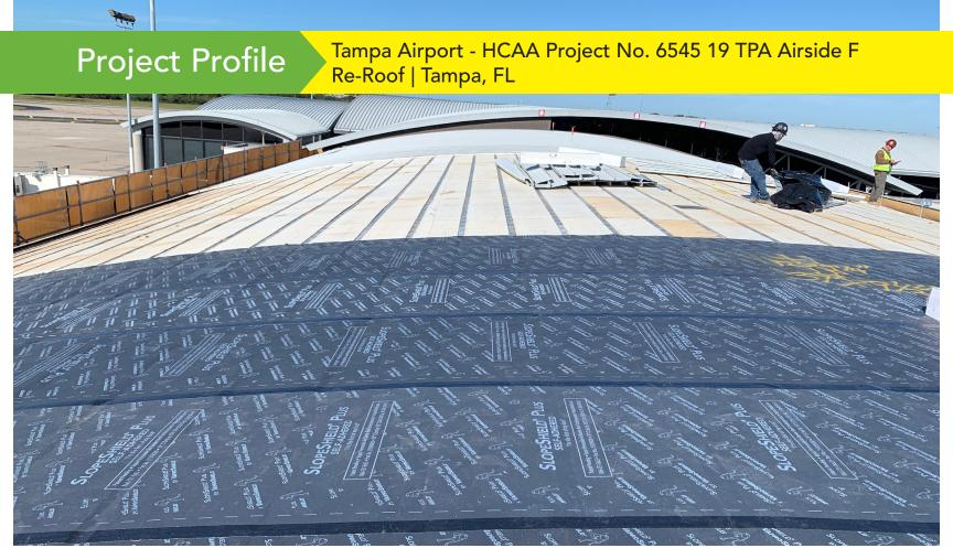
Over 120,000 sq. ft. of SlopeShield Plus Self Adhered was installed over existing roofing materials at the Tampa Airport, HCAA Project No. 6545 19 TPA Airside F Re-Roof. One of the key reasons the Architect chose SlopeShield Plus SA was its **ability to breathe** (due to its permeability), drying any moisture that would occur between the existing roofing material layers.
