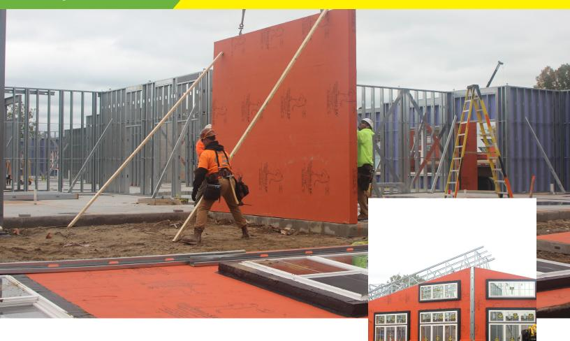
Over 90,000 sq. ft. of WrapShield SA Self-Adhered was installed on prefabricated panels for a state-of-the-art Veteran's Home in Chesterfield, Michigan.
