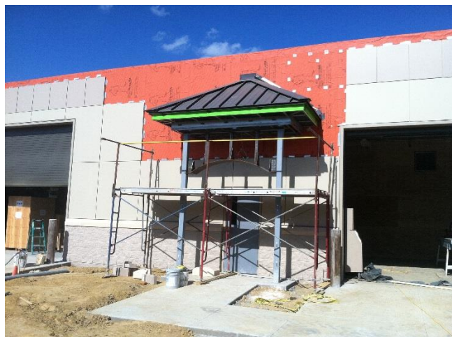
WrapShield SA Self-Adhered offers 6 months of UV and climate exposure protection during installation.
