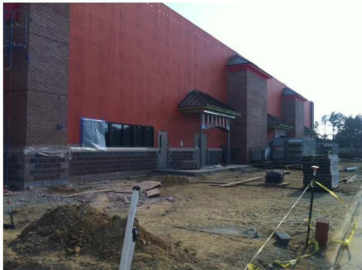
The product was easily applied by the church construction crew.
