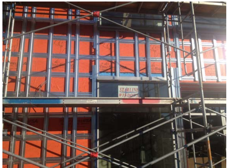
All-weather construction friendly, WrapShield SA Self-Adhered Air Barrier can be installed in temperatures from 20°F (-6°C) and rising, the ideal choice for any climate.
