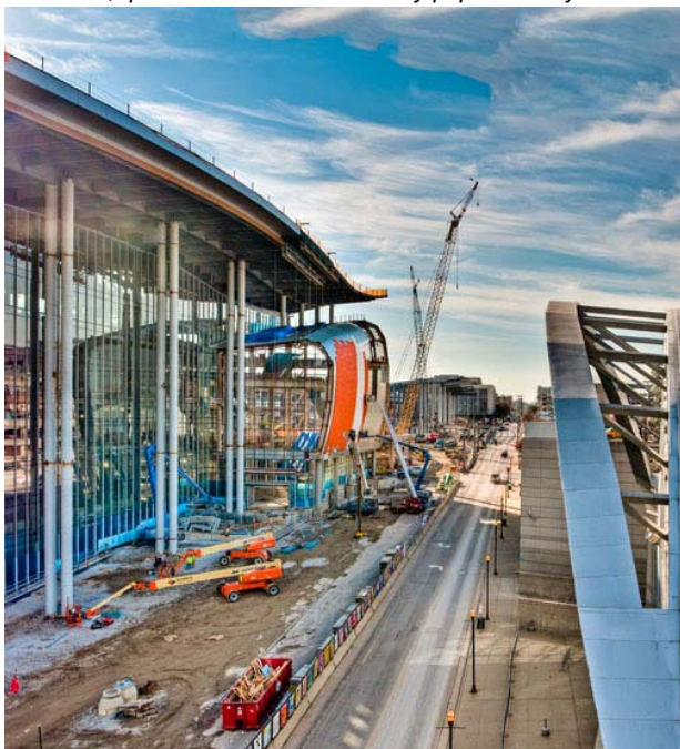
WrapShield SA Self-Adhered (orange) installed over gypsum on the “the drum,” part of the distinctive 5 story pop-out lobby.
