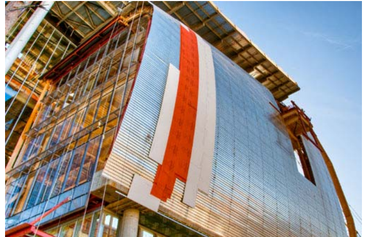
WrapShield SA Self-Adhered (orange) installed over gypsum
